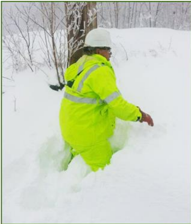
An AEP Transmission line mechanic walks through deep snow ahead of a plow to reach a switching structure.
